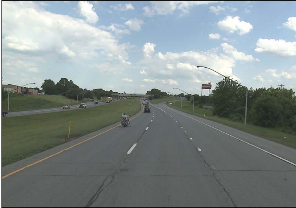
Southbound Travel Lane Typical Pavement Condition
