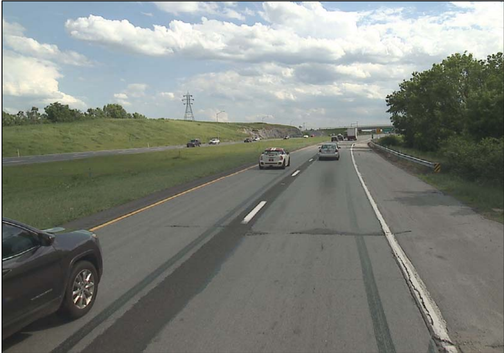
Southbound – County Repairs Longitudinal Joint Patch and Transverse Joint Spray Patching
