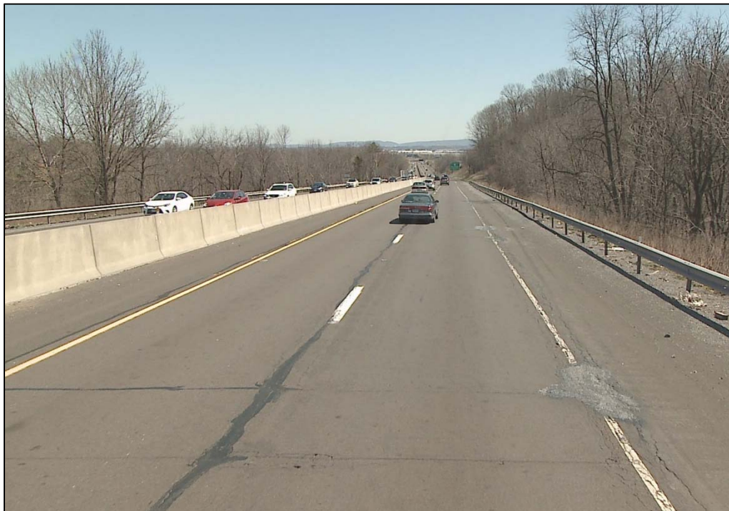
Eastbound Passing Lane – Segment 0470 (Lehigh County) Typical Pavement Condition
